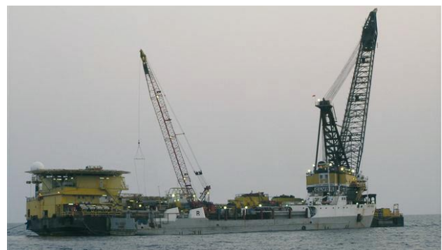
Figure 7. Construction of offshore pipeline.
