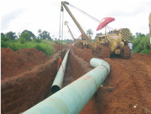
Figure 2. Onshore pipeline construction in Ghana.
