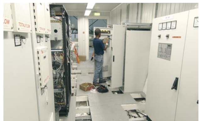
Figure 4. Electrician wiring UPS fault signals to integrated SCADA system.
