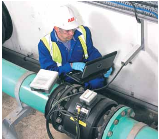
Upgrading electromagnetic flowmeter electronics.
