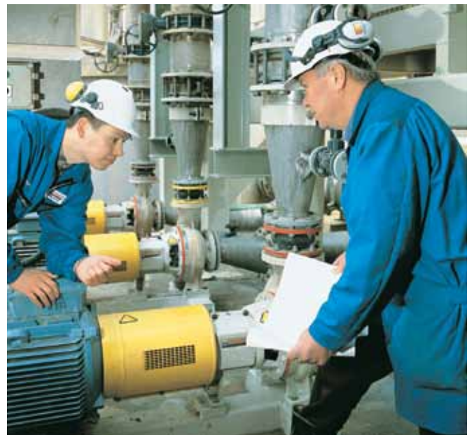
Two ABB drives keep the water flowing at West of Scotland Water's Lomond Street waste water pumping station, Helensburgh, Scotland saving £80,000 in energy over 20 years.
