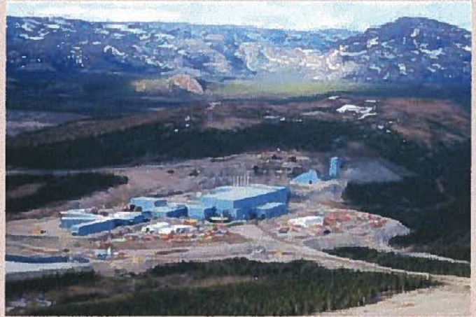
A remote location and lack of local infrastructure contributed to Vale Inco's decision to rely on outsourced services for start-up of a $1 billion greenfield nickel mine and concentrator.
