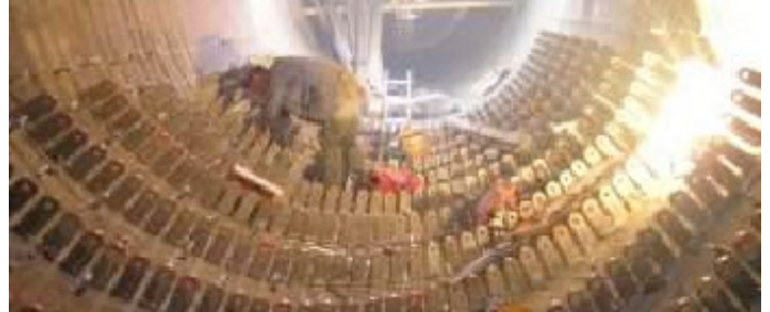
Renewing the chain zone inside of the kiln.
