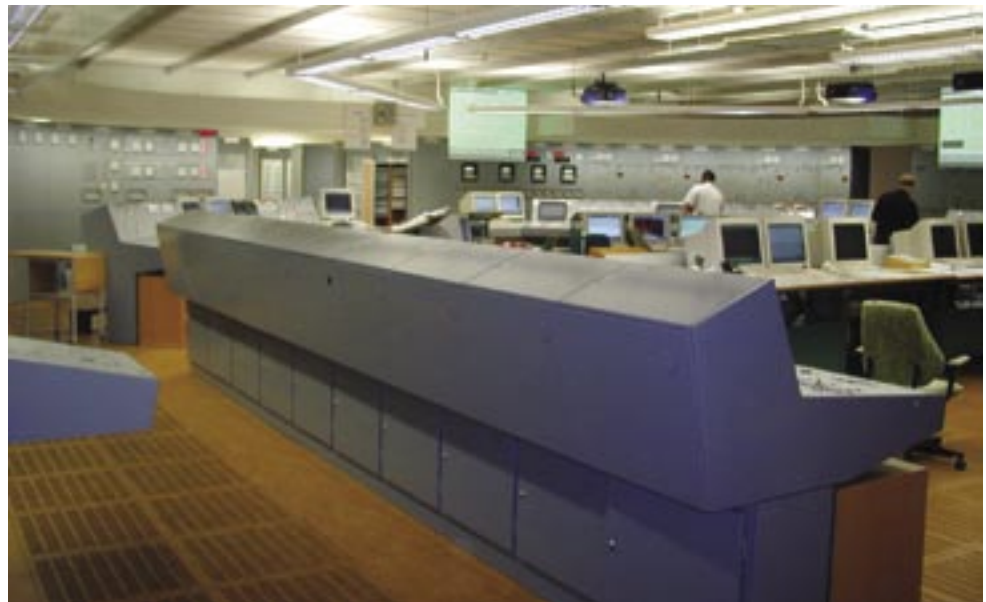
Figure 3. Example of training simulator with identical control room as plant
