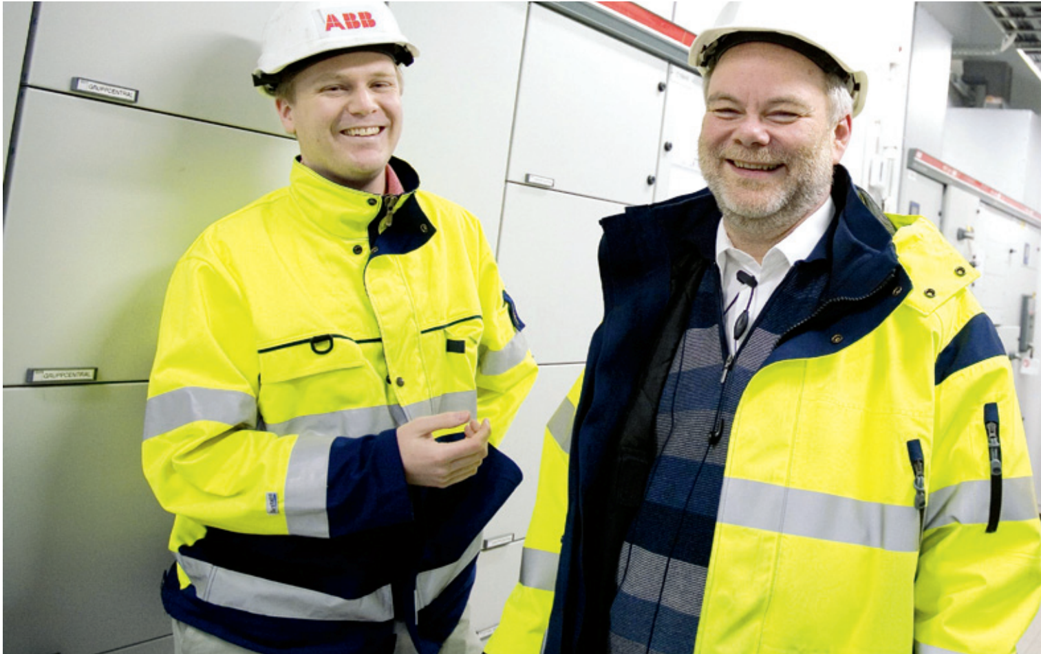
In E.ON's new pumping station in Malmö, the 800xA system also controls a lot of ABB equipment. Here can be seen Henrik Persson, ABB, Torulf Wiberg, Deterministic Control, and Thomas Björklund, E.ON, in front of ABB's low-voltage switching station, MNS Light.
